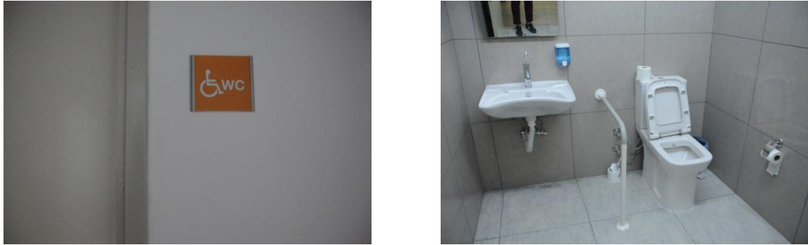
Figure I.2.3.23 Toilet for disabled in the Office Building
