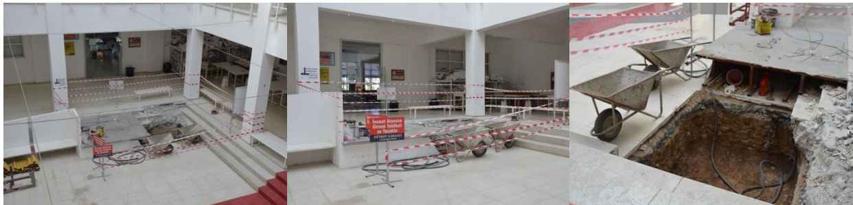
Figure I.2.3.17 Elevator for universal access in the Colored Building in progress
